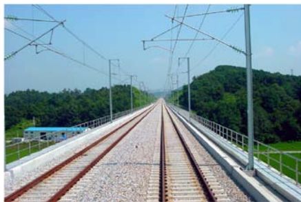
Figure 2 Ballasted HSL track of KORAIL
