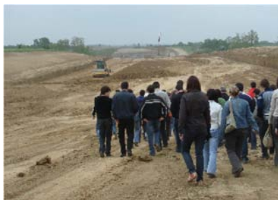
Figure 2 Visit to the Construction Site of a Section of the A5 Motorway, Dakovo, May 2008
