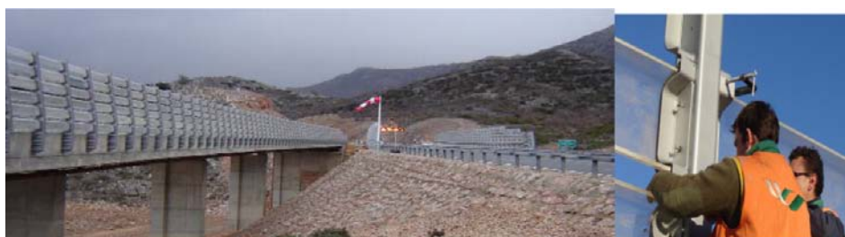
Figure 8 The permeable windbreak structures with transparent panels
