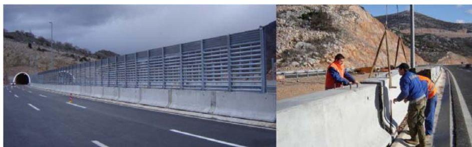
Figure 7 Plate-like windbreak structure
