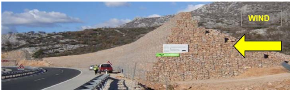
Figure 6 Solid windbreak structures type “high embankment”
