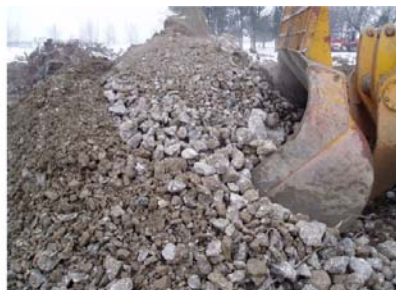
Figure 3 Sopnica-Jelkovec Site: Recycling of Material on Site (a) and Recycled Material (b)
