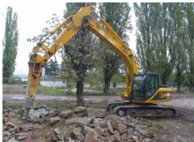
Figure 2 Site II – Špansko-Oranice: Removal of Floor Tiles (a) and Recycling of Material (b)
