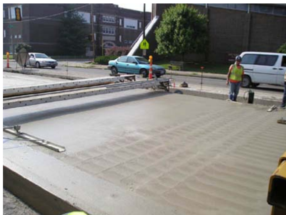
Figure 1 Concrete pavement in the placing stage
