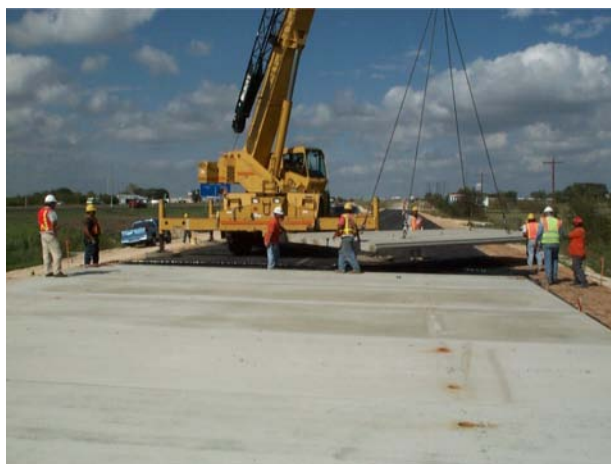
Figure 4 Concrete pavement made of precast elements
