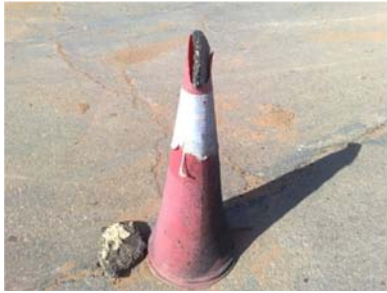
Figure 3 Barriers do not comply with the technical specifications
