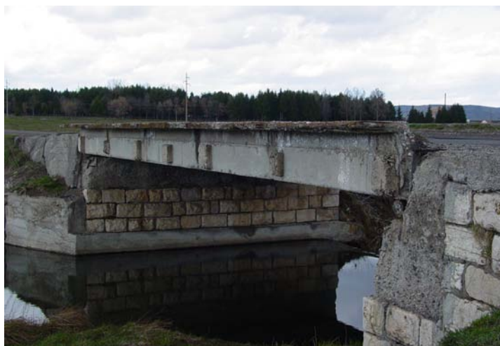
Figure 2 View of existing bridge
