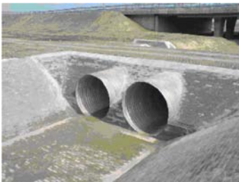
Figure 7 Steel Culvert with Two Spiral Tubes
