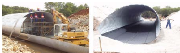
Figure 5 Construction of a Passage on the Vodnjan – Pula-Istria Y Road
