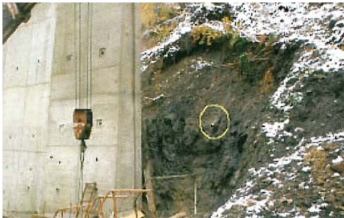
Figure 23 Anchored reinforced-concrete wall with the installed bottom row of anchors
