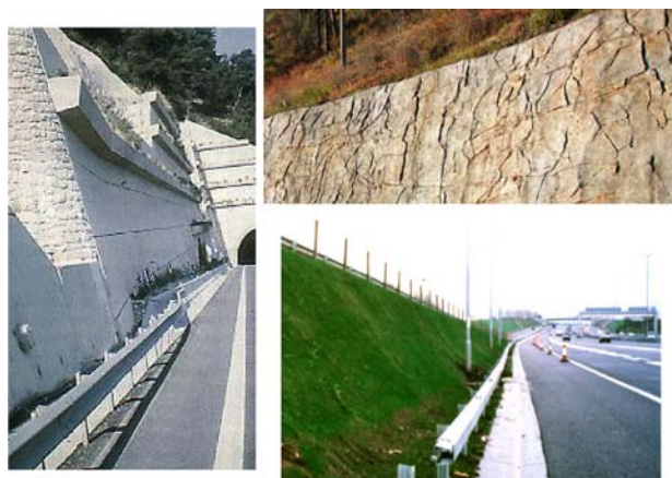
Figure 4 Various types of soil nailing facing finishes: precast face panels (left), shotcrete facing styled as rock outcrop (top right), panels with vegetation growth (bottom right)
