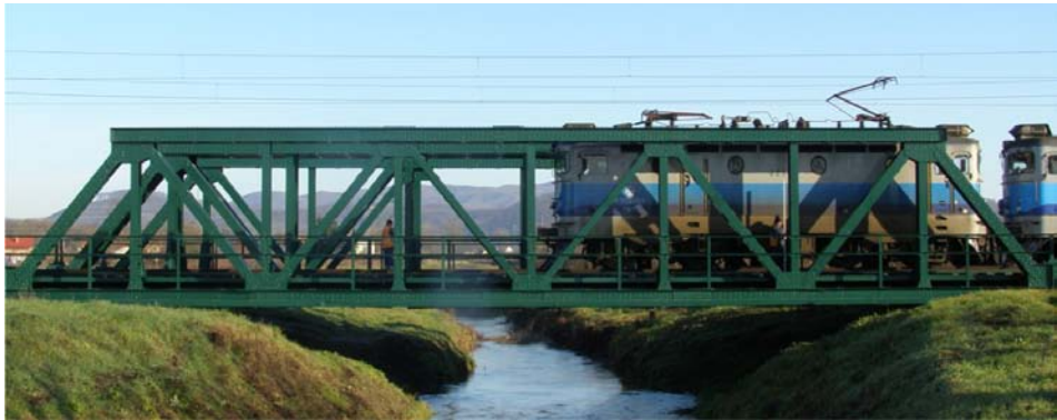
Figure 1 Front view of the steel truss bridge (north-upstream)
