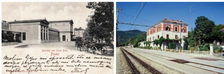
Figure 6 The second railway station in Rijeka built in 1890 (left) and railway station in Matulji, built in 1883 (right)
