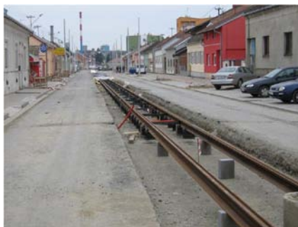
Figure 8 Placement of tracks on provisional support
