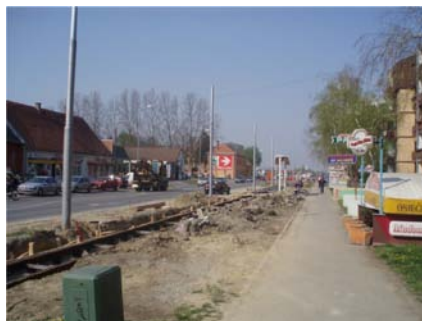
Figure 5 Building of tram tracks
