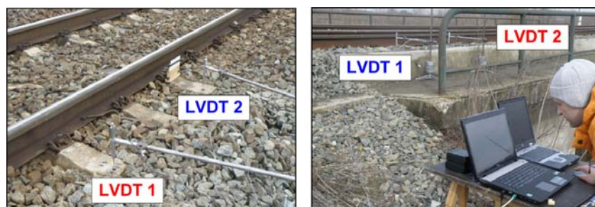
Figure 12 Results of measurement (left km 0+371, right km 5+938-bridge “Dren”)
