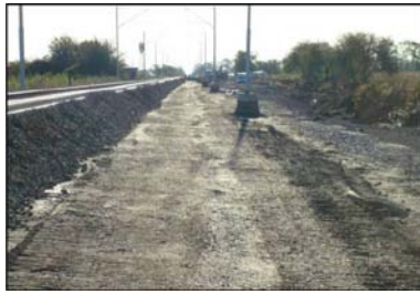
Figure 2 Works at the planum level
