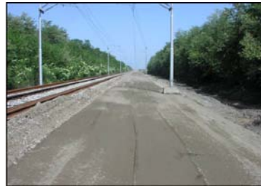
Figure 3 Works at protective layer level
