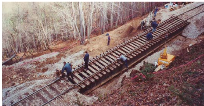
Figure 8 Temporary improvement measure
