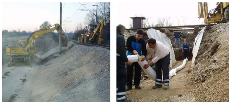
Figure 6 Execution of transversal drainage ribs
