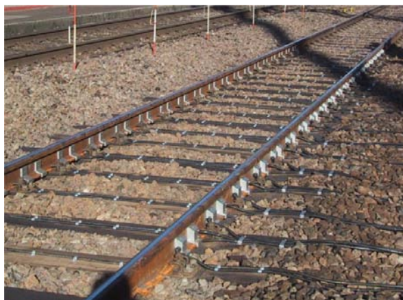
Figure 5 ARGOS Level 2 on wood sleepers
