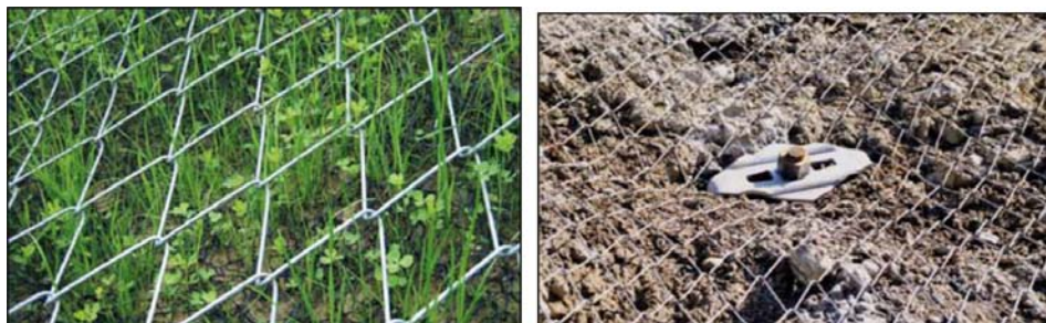
Figure 1 High-tensile wire mesh for slope stabilization (left) and special spike plate to actively pressing the high-tensile steel wire mesh against the slope surface (right).
