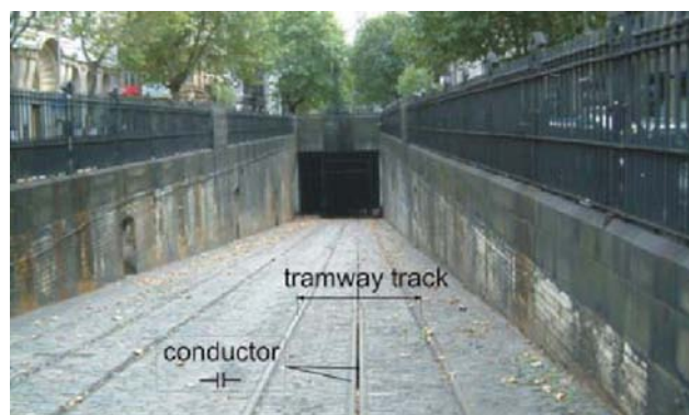
Figure 1 Kingsway Tramway Subway, London – north entrance, 2003, [4]
