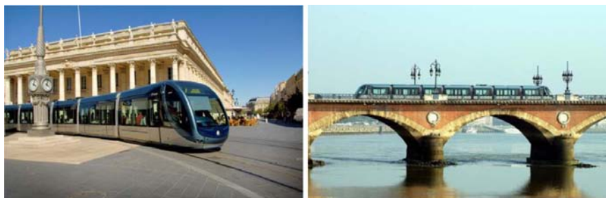
Figure 5 Citadis and APS in Bordeaux (square, bridge) [13]
