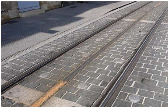
Figure 3 Third rail of APS, Bordeaux
