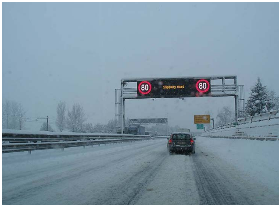
Figure 1 Winter conditions on a highway. [Source: cgs plus d.o.o.]
