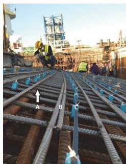
Figure 4 Topology of corrosion protection techniques
