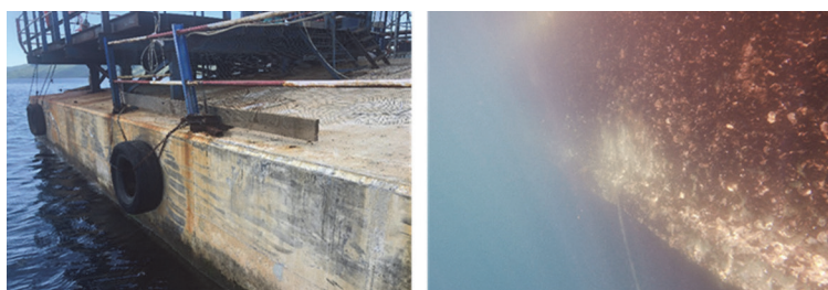
Figure 3 Pile caps above and below the water line
