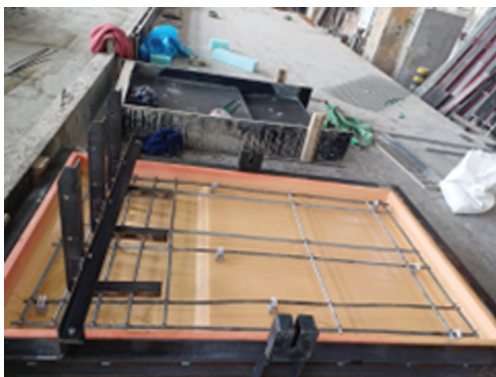
Figure 4 The silicon molds of Bridge kerb elements
