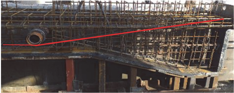
Figure 2 The steelstructure and the strainline marked with red line
