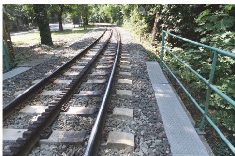
Figure 3 A photo of the track of Budapest Cogwheel Railway
