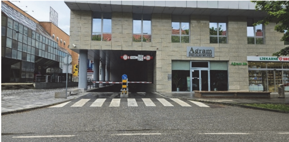
Figure 1 Entrance to the garage in Istarska Street
