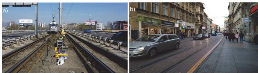
Figure 3 Track with discretely fastened rails: a) opened and located in separate band, b) closed and built as part of the road surface
