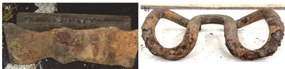
Figure 5 Sample of corroded rail and clip taken from urban track infrastructures
