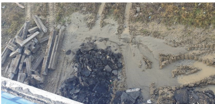
Figure 3 Sand extrusion from a soil crack near pier S4 [2]
