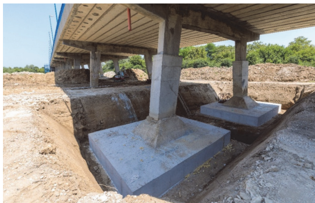
Figure 5 Widening and strengthening of bridge piers
