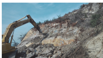
Figure 2 Soft rock environment at the widening of the main road 21, Hungary
