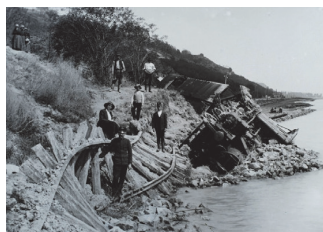
Figure 3 Railway accident caused by landslide on the shore of Lake Balaton in 1914 [10]
