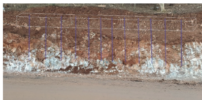
Figure 10 Landslide rehabilitation with horizontal beam
