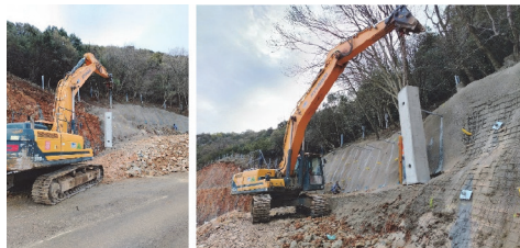
Figure 9 Placing beams on previously constructed anchors
