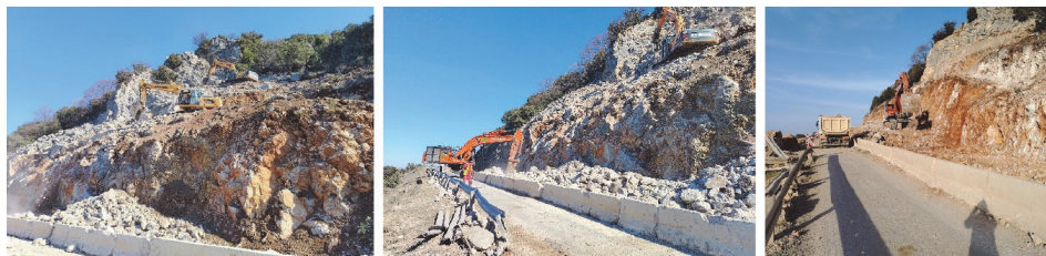
Figure 6 Work on ramp construction
