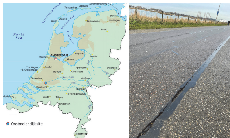
Figure 2 Oostmolendijk location & example of observed deformations and cracks
