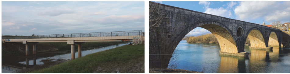
Figure 1 Case studies: Kučki Bridge (left) and Kosinj Bridge (right)
