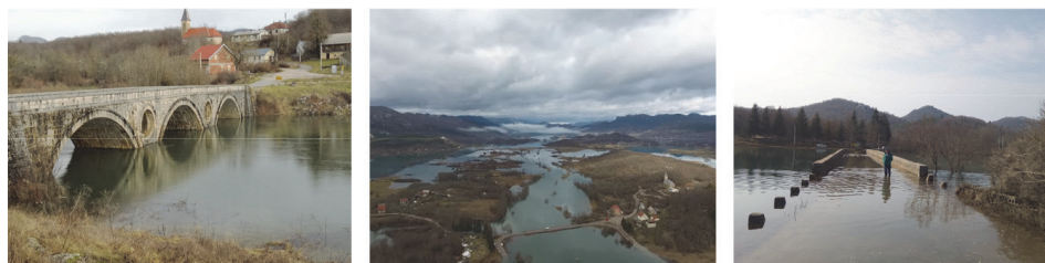
Figure 6 Kosinj Bridge during high water levels of the River Lika
