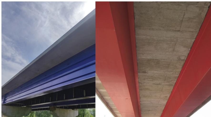
Figure 1 Composite bridges with open (left) and closed (right) cross-sections of the main girder
