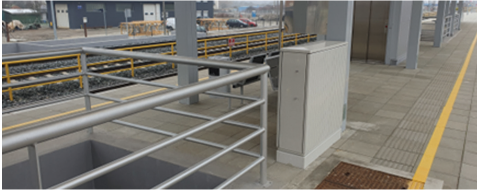
Figure 2 Field inspection – grouping multiple fixed objects
