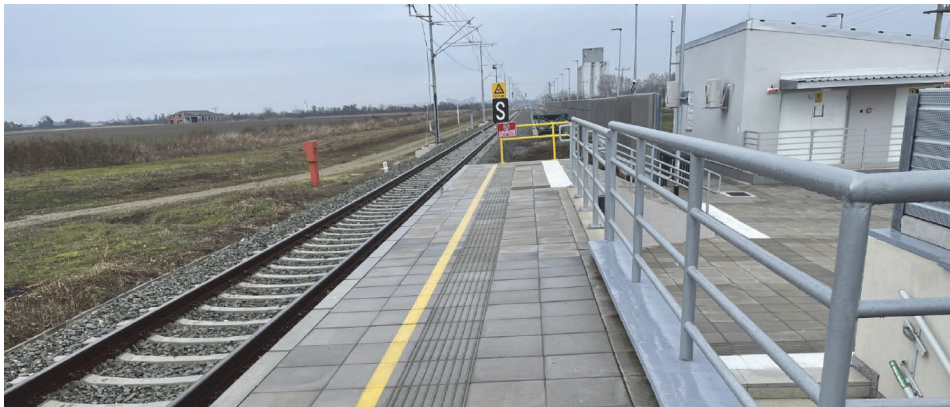
Figure 3 Field inspection – platform of insufficient width
