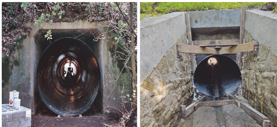
Figure 1 Examples of relining applied in a railway structure
