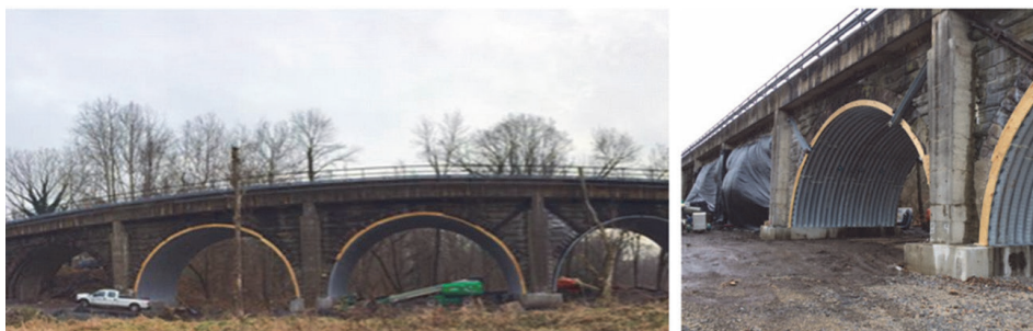
Figure 2 Strengthening of stone vaults
