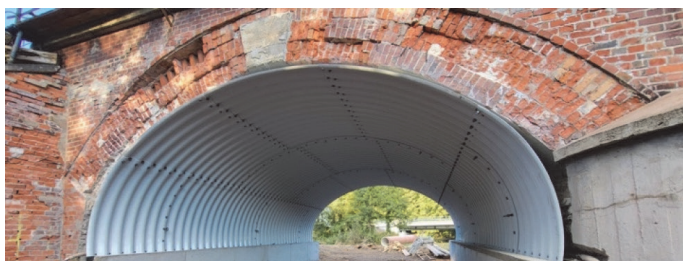
Figure 7 Example of the facade during strengthening of a masonry vault
