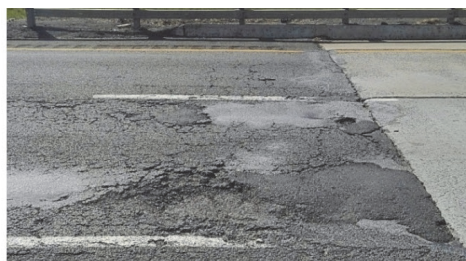
Figure 8 Axle detection sensor and damaged pavement at the bridge approach
