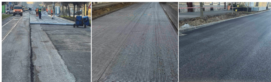
Figure 5 The reinforcement mesh on the prepared base and laid asphalt layer
