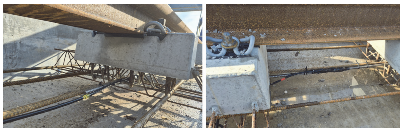
Figure 4 Sensors installed on the test section in Sarajevska road
