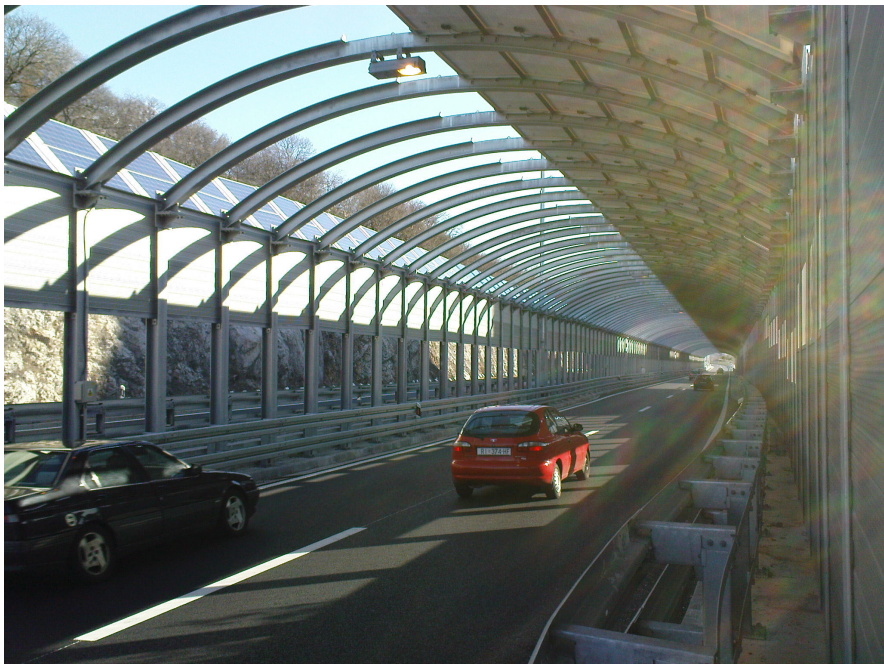
Figure 4 Constructed integral system – view from inside.
