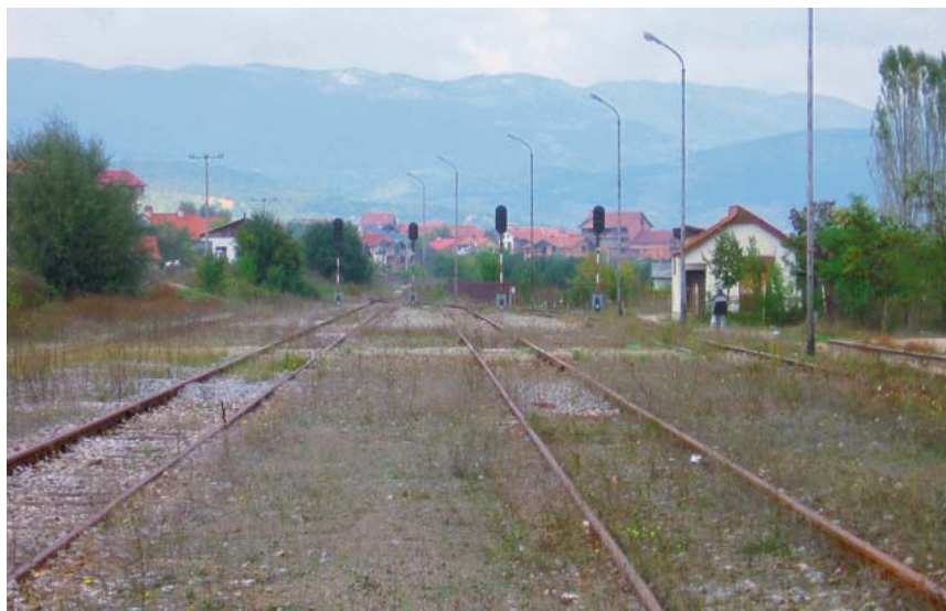
Figure 6 Kicevo Station: terminal of the existing railway line towards Albania
