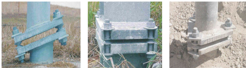
Figure 14 Examples of the break-away NE columns [4]
