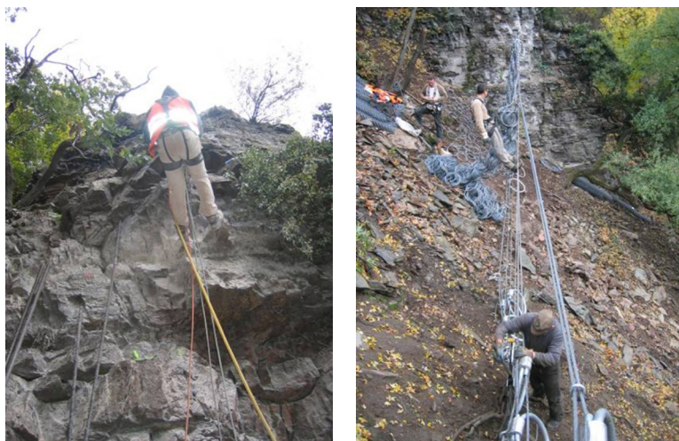
Figure 5 Drilling being carried out on ropes (left) and fixing of the ring net after the installation of support ropes (right).
