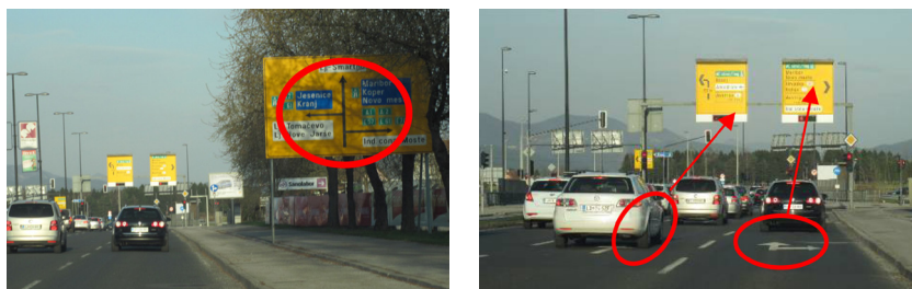
Figure 3 Clear: Does the driver know what to do? Which direction? What lane? Are the signs and lane markings correct? Does the driver have all the necessary information? Traffic signs among themselves and with road markings are not consistent.
