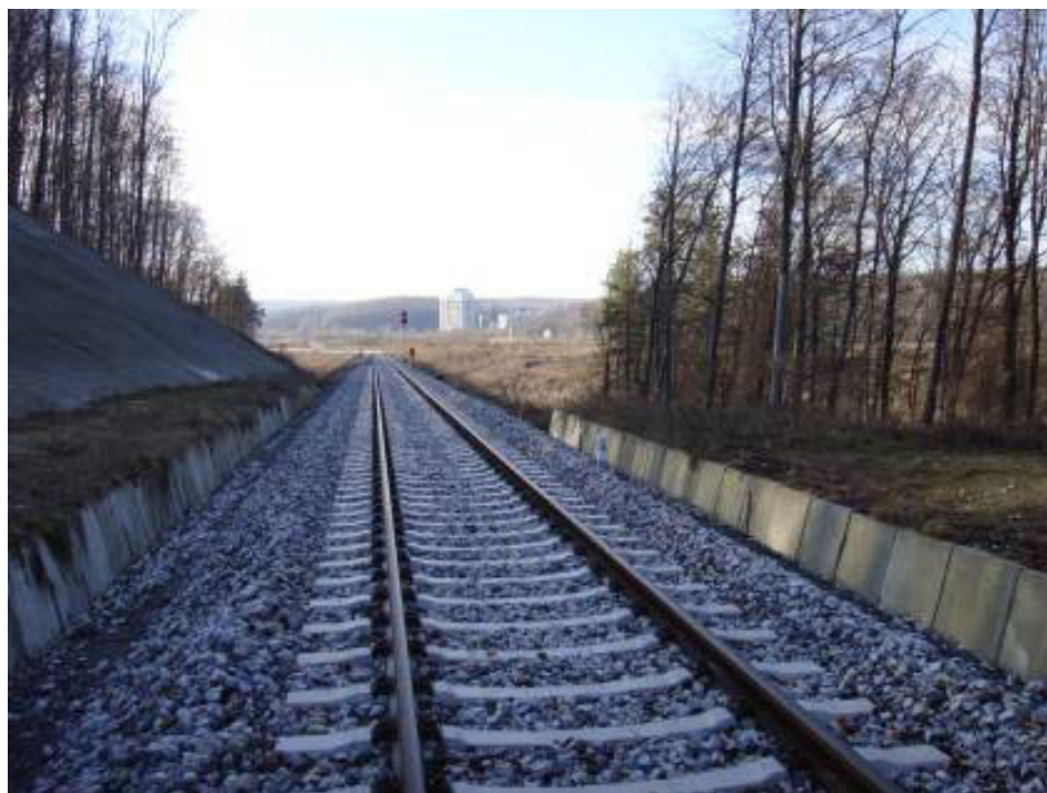
Figure 4 Special track of cement factory Našicecement
