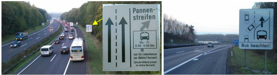
Figure 6 Road signs to indicate that regular service buses are permitted to use the emergency lane (text on the left: emergency lane ... Mon.-Fri. 6:00-9:00 a.m. ... only for public buses to exit Dornach (text at the bottom in Czech) text on the right: Watch for buses!)
