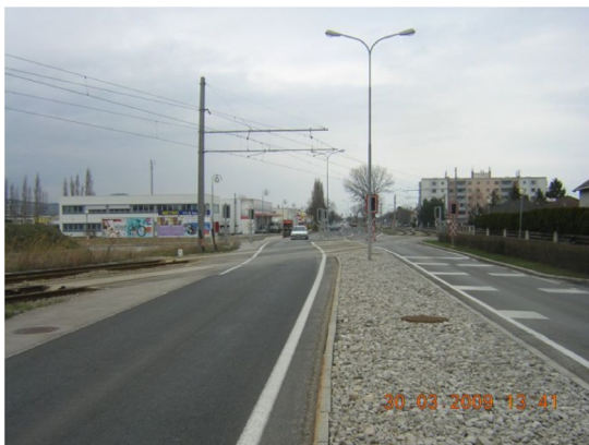
Figure 8 Two-track light rail changing sides of a road (Badener Bahn at LB17, Traiskirchen, Austria). Photo: T.Brezina.
