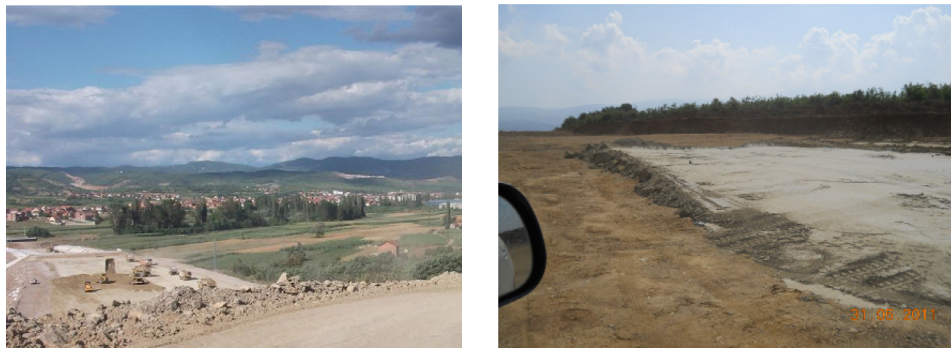
Figure 6 View of the beginning of embankment construction with material from cutting, which was to be used as material category C, and a view of the test field where it was confirmed that this material is not to be placed in the embankment without improvement.
