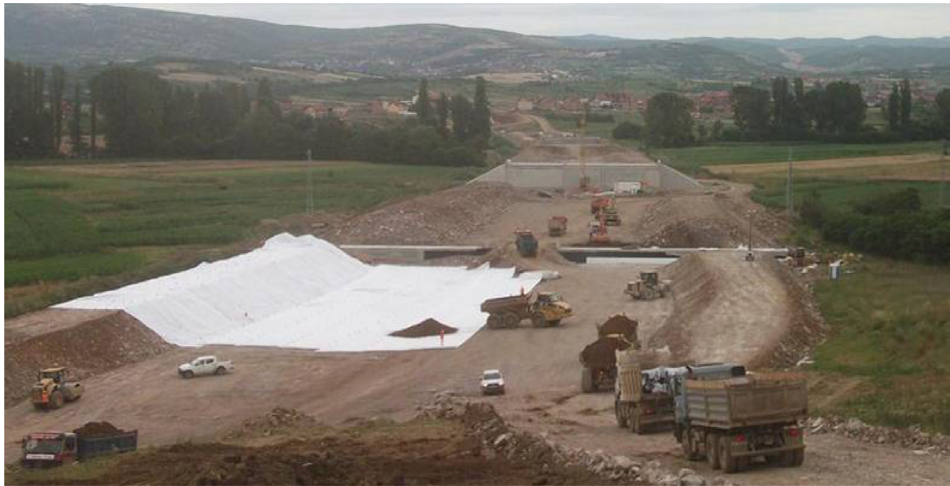
Figure 8 Construction of layers of large embankment covered with geotextile.
