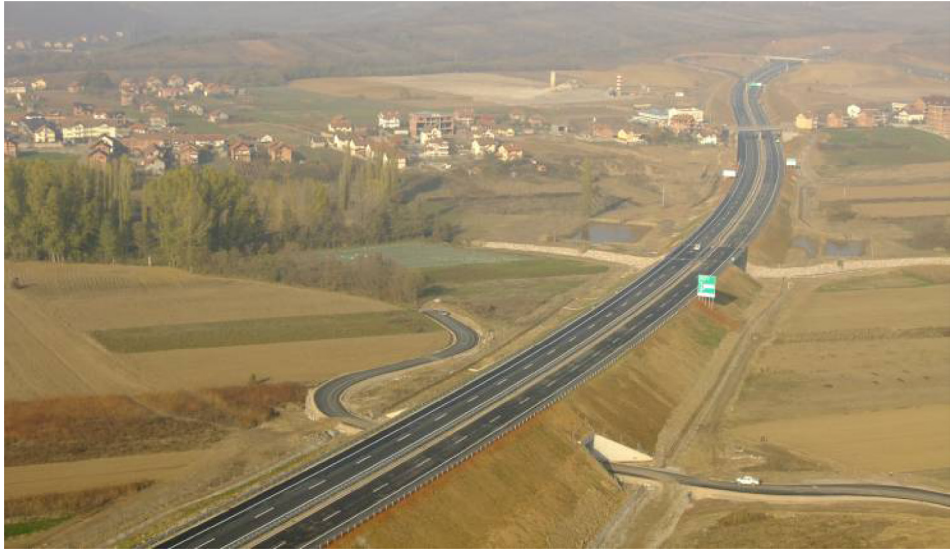
Figure 11 Completed motorway on the large embankment part.
