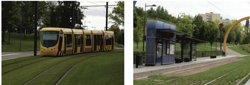
Figure 5 Perfect green track (left) in Mulhouse and the damaged green track at a terminal stop (right) caused by (too) long idle time and multiple mechanical impacts by trespassing passengers
