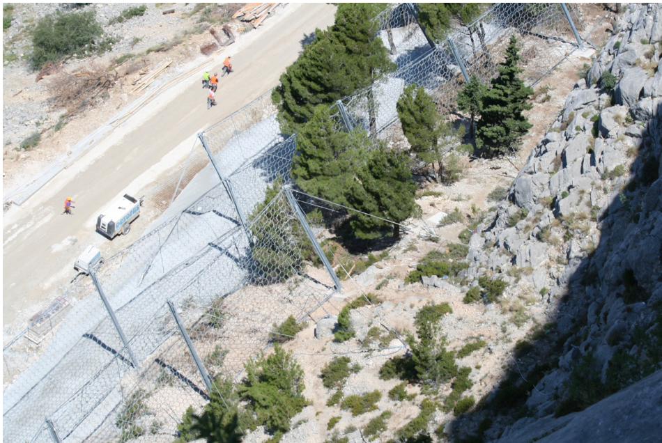
Figure 6 Constructed barriers Retaining unstable boulders
