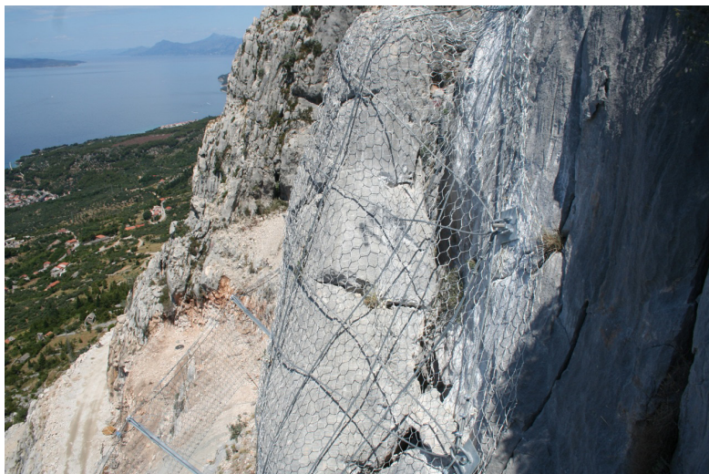
Figure 7 Retaining unstable boulders
