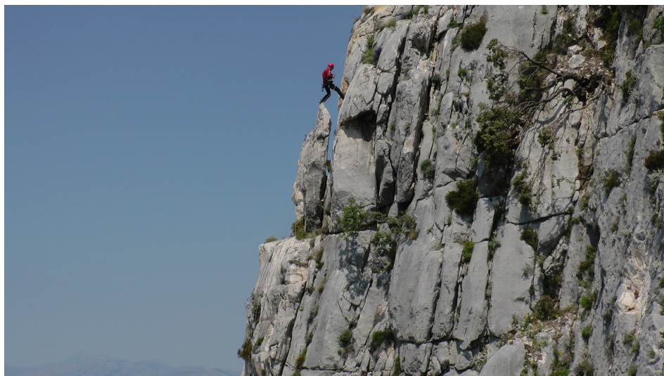
Figure 4 Unstable boulder no 41 located using geological–alpinist mapping
