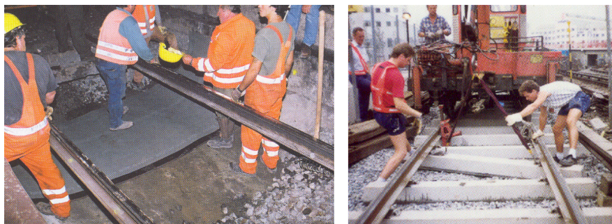
Figure 1 Additional building in the under ballast mats and the sleeper pads
