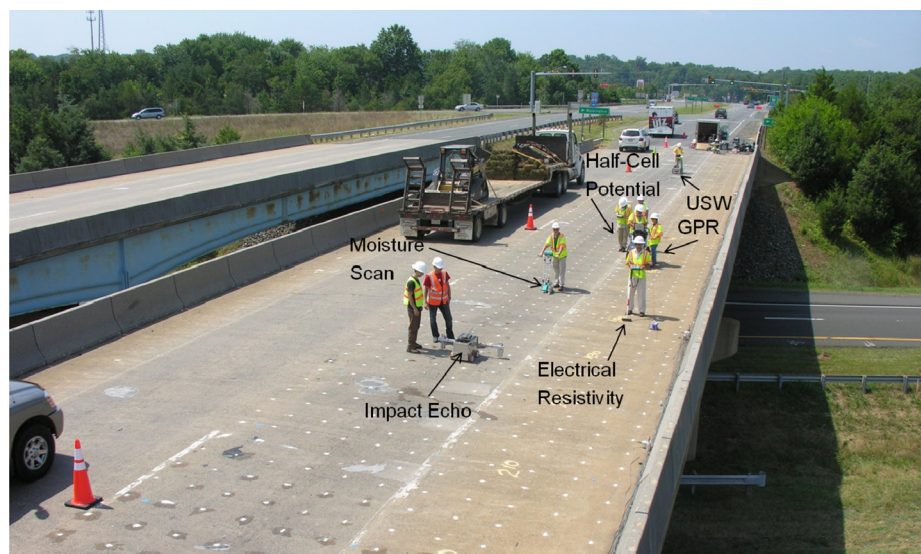
Figure 4 NDE survey of a bridge in Virginia.
