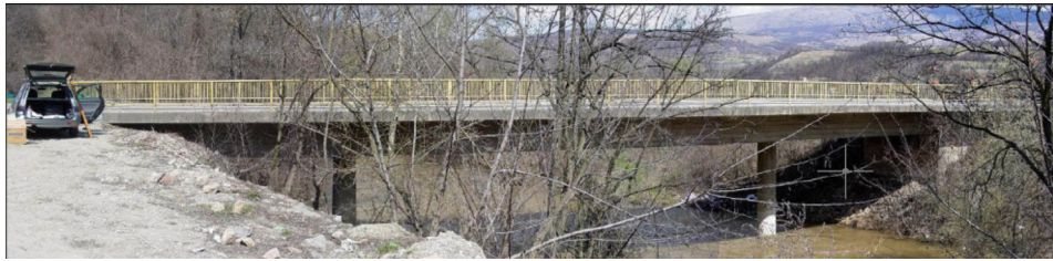
Figure 1 Upstream view of the existing bridge
