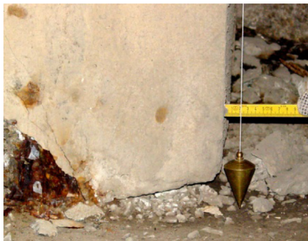
Figure 2 Vertical impairment and deviation of bearings
