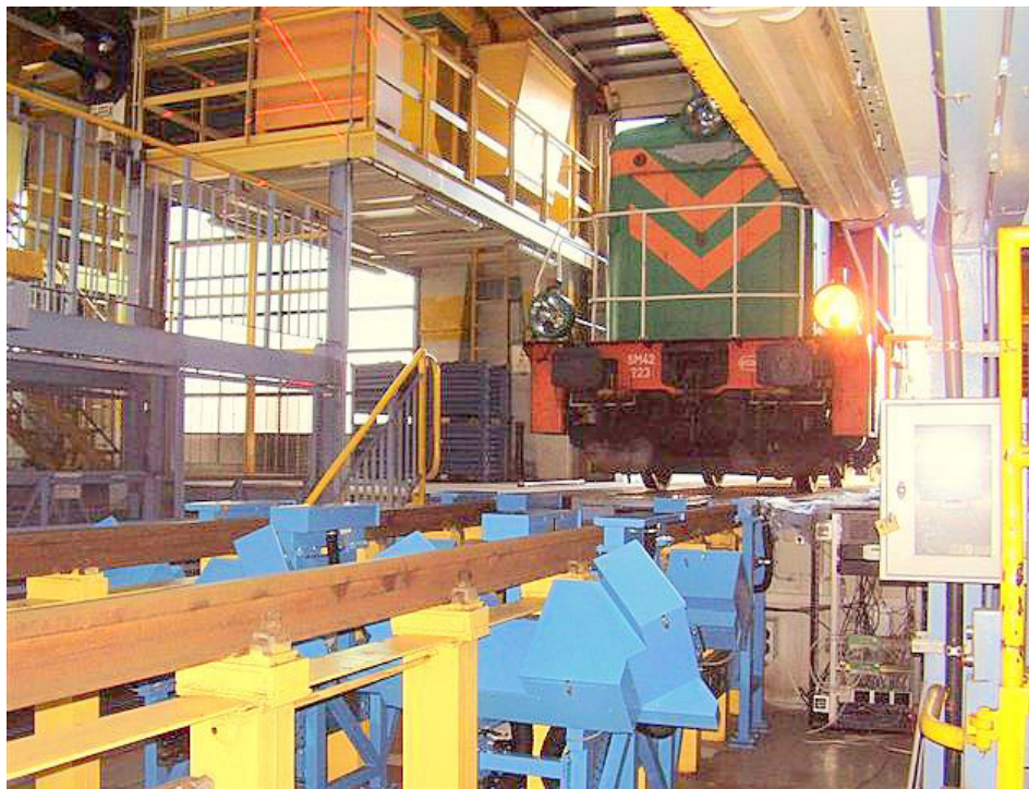
Figure 1 Train entering the measurement system at Intercity Depot in Warsaw
